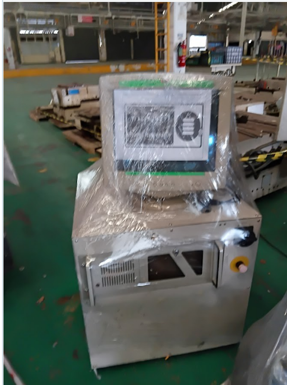
Computer and operator station
